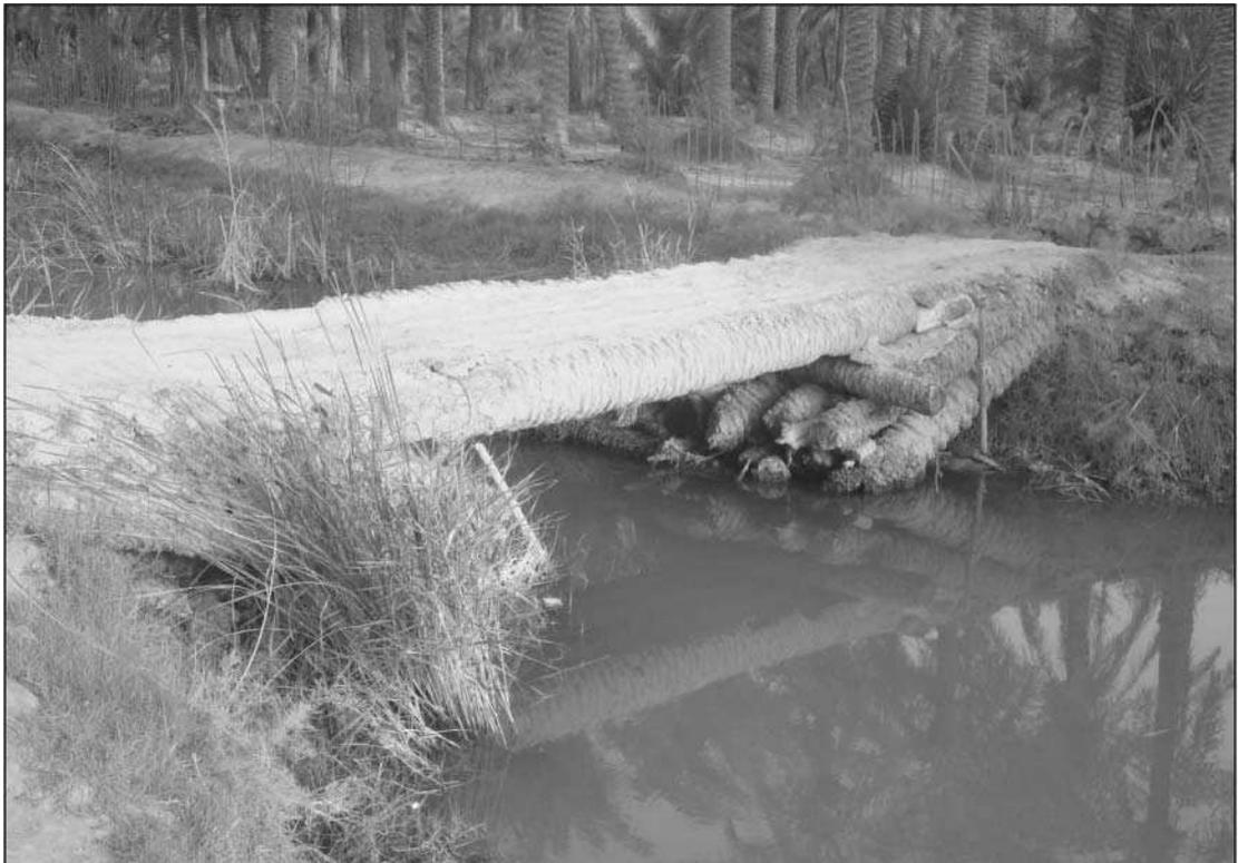
Fig. 7 Regulator/palm-tree bridge at the Umma Nakhlah canal (a side branch of the Euphrates river) south of Suq ash-Shuyukh, photographed by Abdulamir Hamdani, 2010.
